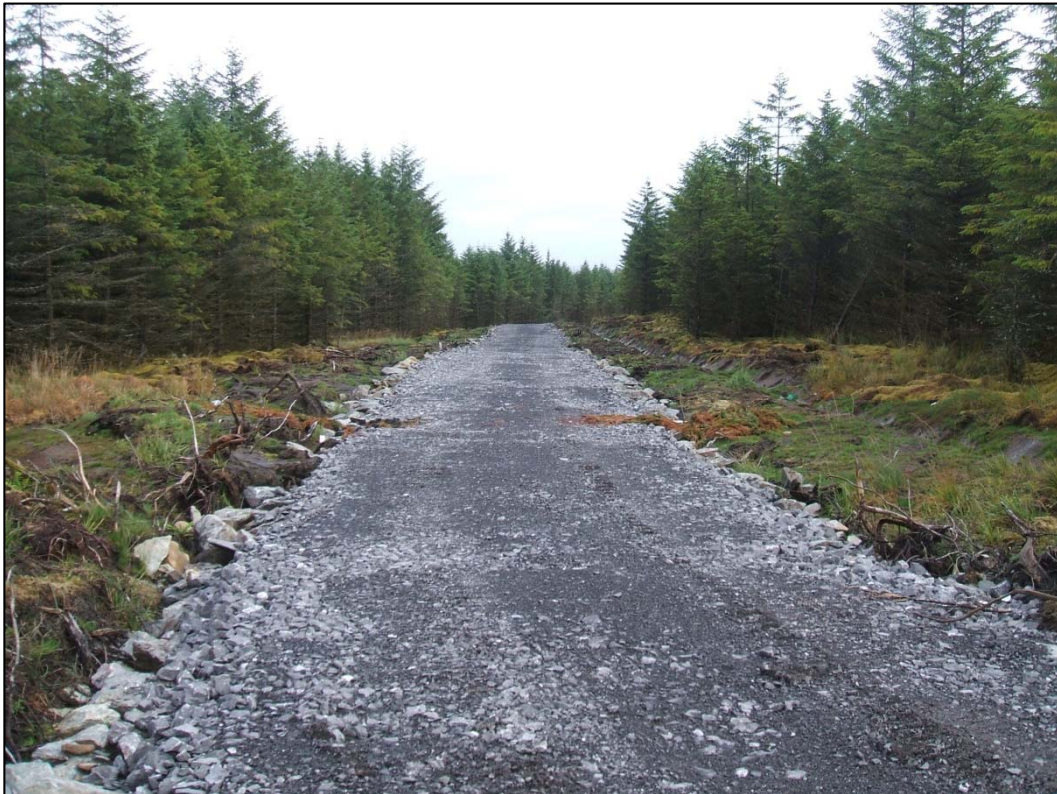
Photo 4 Example of an existing floating access track on site
