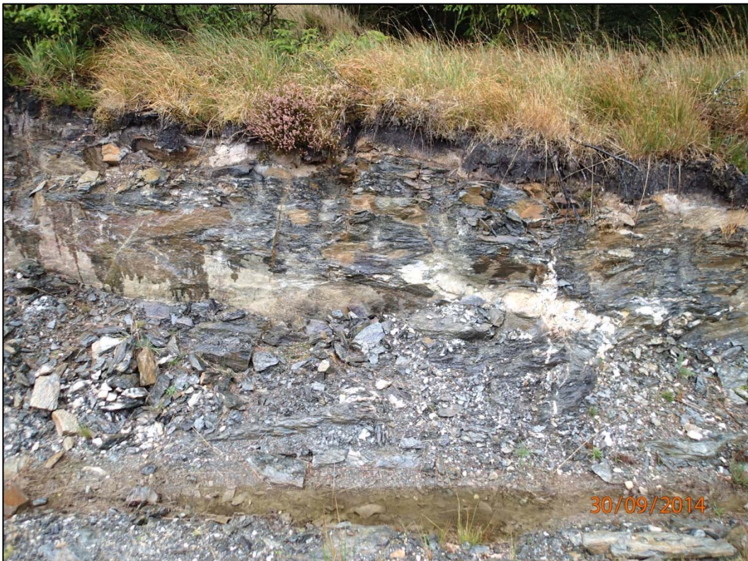
Photo 6 Example of ground conditions on site (shallow peat area)
